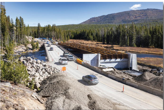
Lewis River Bridge replacement: girders and south abutment. NPS / Jacob W. Frank
